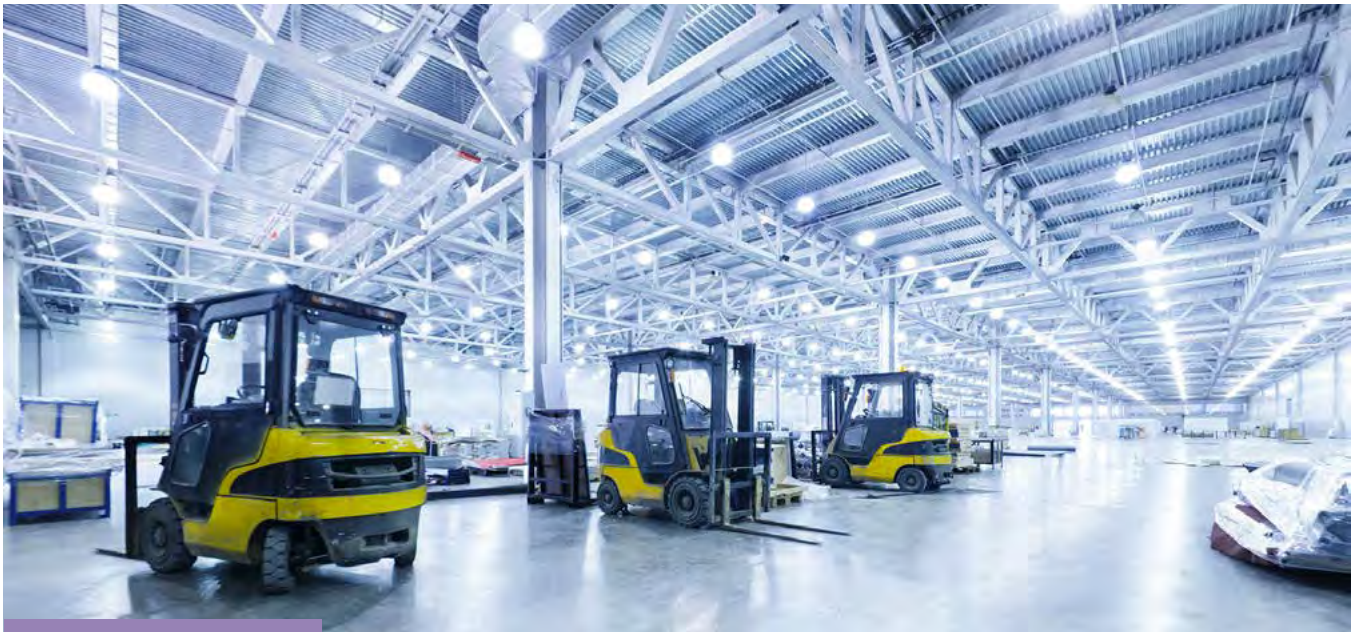
LED lighting in a warehouse
