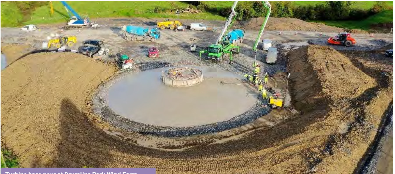
Turbine base pour at Drumlins Park Wind Farm
